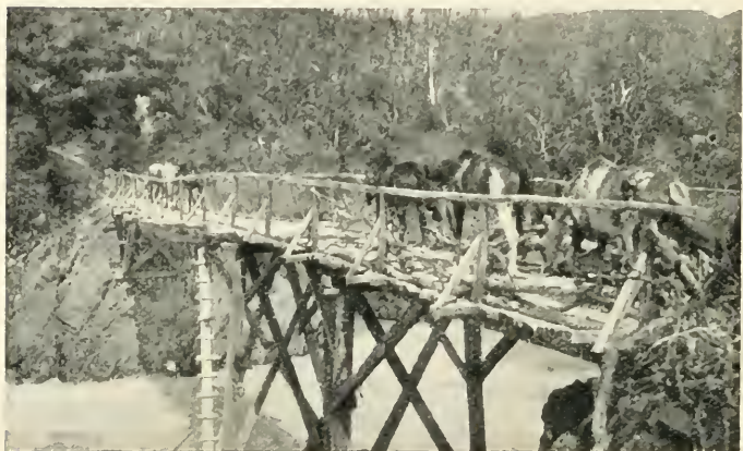
BRIDGE OVER RIO DEL SALTO, PATAGONIA.
